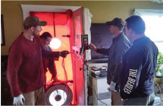
Blower door testing by the Weatherization Crew
